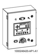
DSE-7420 is an advanced control module based on micro-processor, containing all necessary functions for protection of the genset and the breaker control. It can monitor the mains supply, and automatically start the engine when the mains is abnormal. Accurately measure various operational parameters and display all values and alarms information on the LCD. In addition, the control module can automatically shut down the engine and indicate the engine failure.
